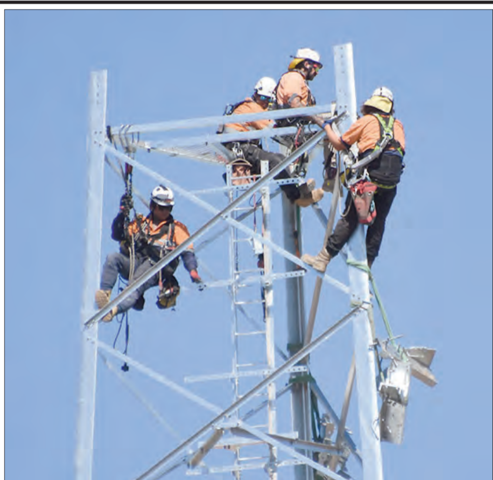
• Four brave men at the top of the new Optus tower.
